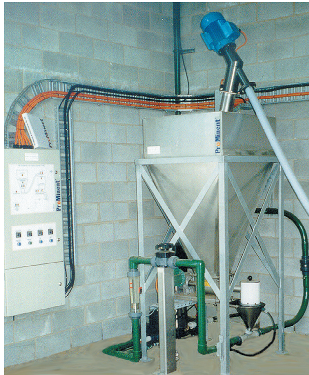
Powdered Activated Carbon Preparation System
